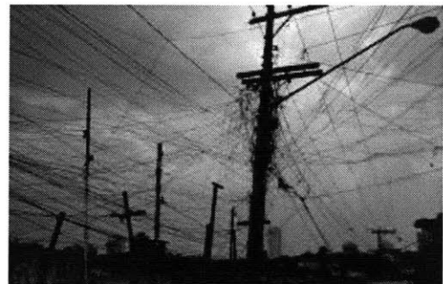
Figure 3: Example of electricity theft in a Brazilian slum 12
